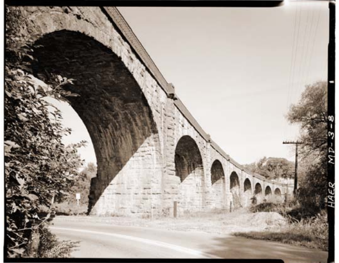
1970 photo looking north at the east side of viaduct from Levering Avenue. From the HAER collection.
