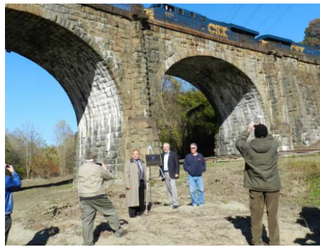
Tod Echler, CSX Chief Engineer for Maintenance, and ASCE President Andrew Herrmann with plaque at base of viaduct as train passes overhead.
