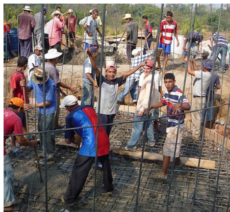
Constructing the water holding tank.
