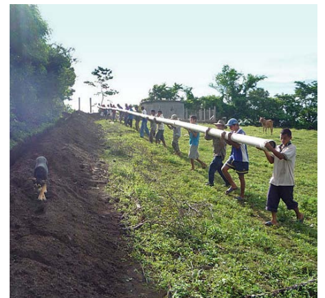
Constructing the water pipeline.
